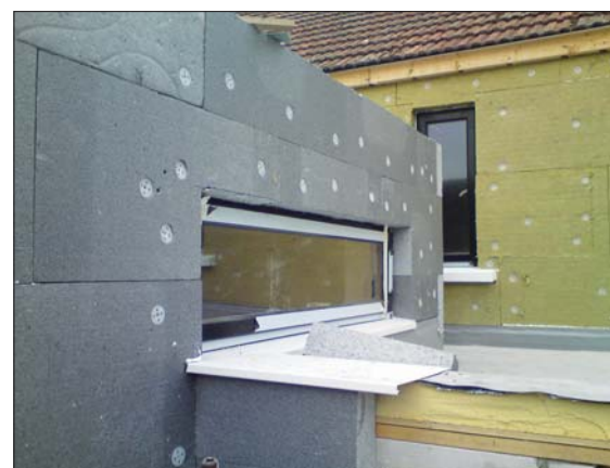
(top) Architect Bobby Conroy specified the Isover Vario airtightness system throughout the build; (above) Quinn Lite aerated concrete blocks were used for new sections of the house; (below) the rear extension is externally insulated with a 120mm Powerwall platinum EPS system while the existing walls are insulated with 120mm high density Rockwool; (left) the house is now divided into four separate heating zones that can be monitored and controlled for maximum efficiency; (p57) the new rear extension houses a bright and spacious kitchen and dining space with underfloor heating
