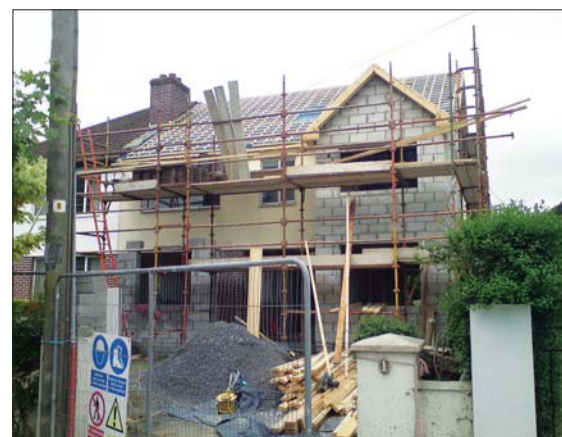
(top) Architect Bobby Conroy specified the Isover Vario airtightness system throughout the build; (above) Quinn Lite aerated concrete blocks were used for new sections of the house; (below) the rear extension is externally insulated with a 120mm Powerwall platinum EPS system while the existing walls are insulated with 120mm high density Rockwool; (left) the house is now divided into four separate heating zones that can be monitored and controlled for maximum efficiency; (p57) the new rear extension houses a bright and spacious kitchen and dining space with underfloor heating
